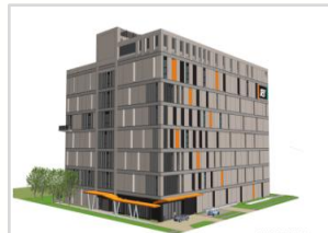
Kaohsiung 3 rd Factory (under construction)
